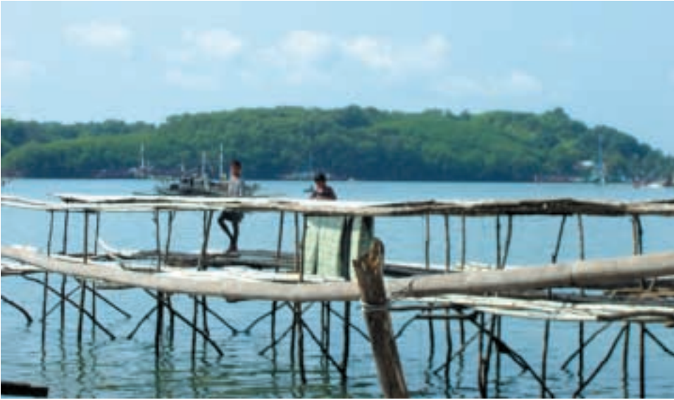
The scaffolding and catwalk of Project Hope in barangay Sangali: the “groundwork” for the Bajao’s community on the sea
